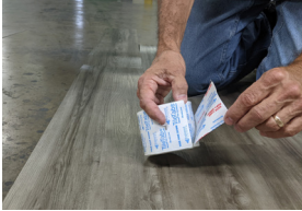
A.1 Peel the TileTab from the roll
