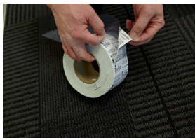
A.1 Peel the TileTab from the roll
